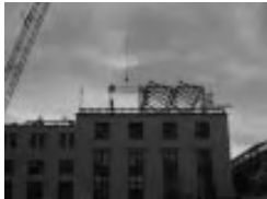
4 day erection process
