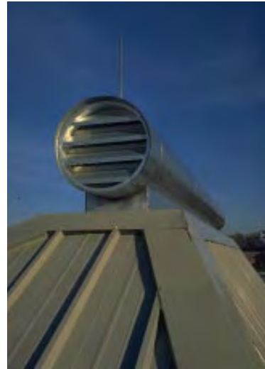
Rooftop ventilators for stack-assist ventilation
