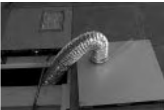
Modular, reconfigurable ducting with tether connections to individual air diffusers
