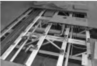
Modular, reconfigurable ducting with tether connections to individual air diffusers
