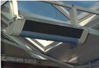
LTG Coolwave™ ceiling-mounted cooling units
